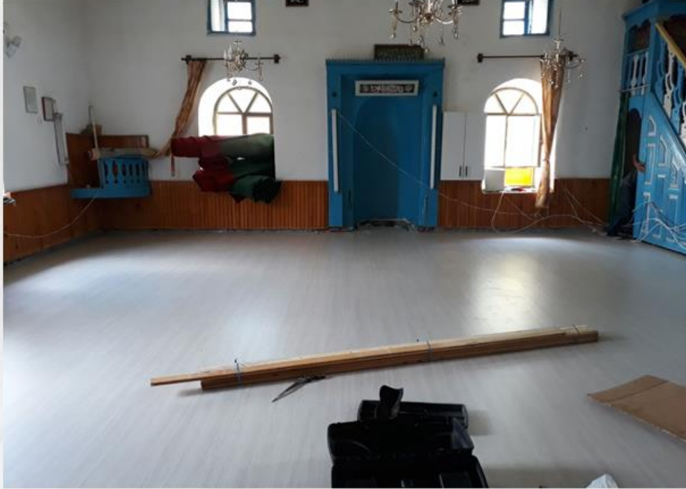
KARAHALİLLER MAHALLESİ CAMİİ LAMİNANT YAPIMI
