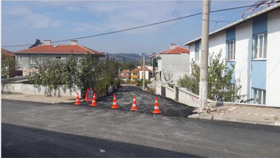
YENİCE MAHALLE HİLAL SOKAK ASFALT YAPILMASI
