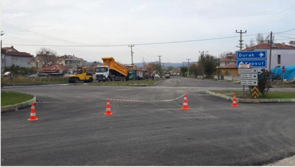
YENİCE MAHALLE ZAMBAK SOKAK ASFALT YAPILMASI
