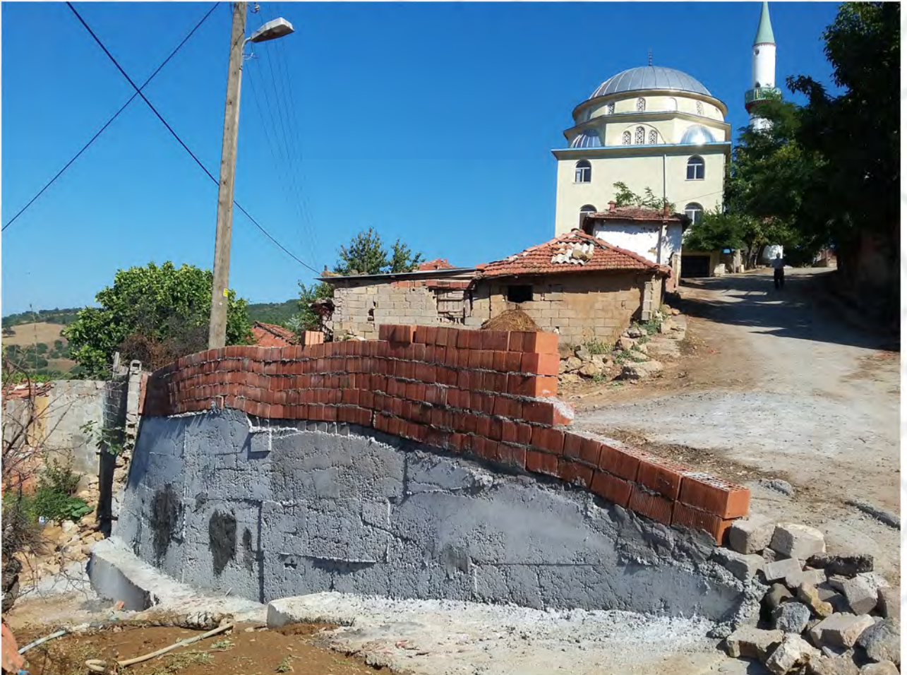
ÖRENHARMAN MAHALLESİ İSTİNAT DUVARI YAPILMASI
