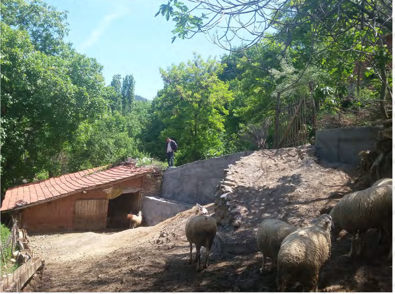
ÖRENHARMAN MAHALLESİ İSTİNAT DUVARI YAPILMASI 1
