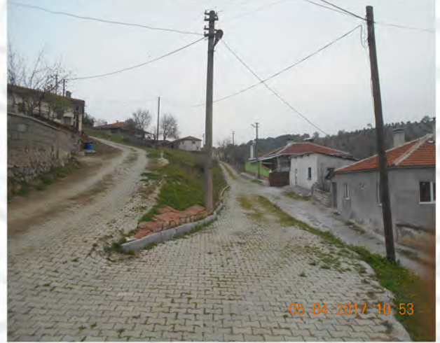
RECEPKÖY PARKE TAŞI YAPILMASI
